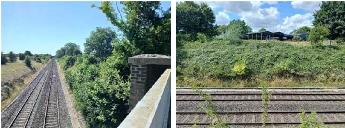
View SE from Raghose Lane Bridge. Scrub S78 to right of frame, Grassland G38 to left. Bramble thicket centrally within scrub S78.
