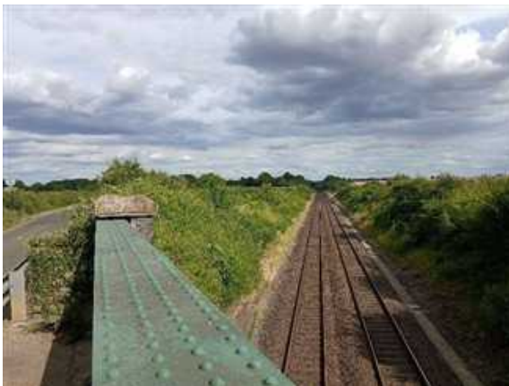
Scrub S80N at start of section, viewed SE from Sommerton Road bridge.
